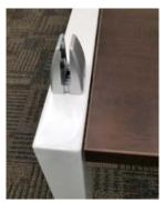
2) Determine what material you are installing. If it is sound-dampening EzoBord you will not need the rubber inserts (pictured below) that go on both sides inside the bracket
